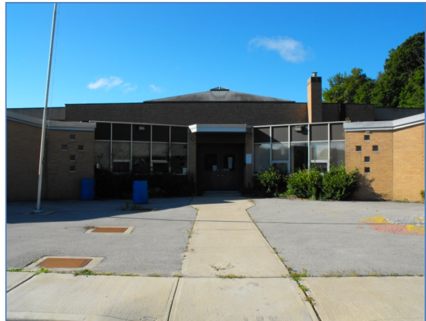
Figure 9 Former Holy Name School
